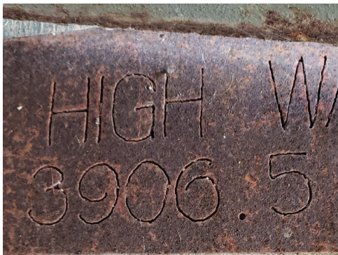
High Water Mark inside Dam 3906.5 ft. Above Sea Level
