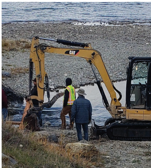
Flathead Indian Irrigation Project "Illegal" Backhoe/Work
